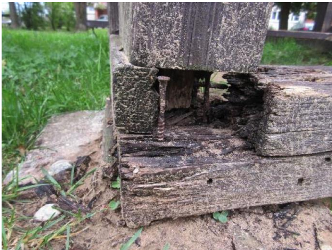
Photograph 7 Example of damage that may lead to collapsing/breaking down of the equipment
